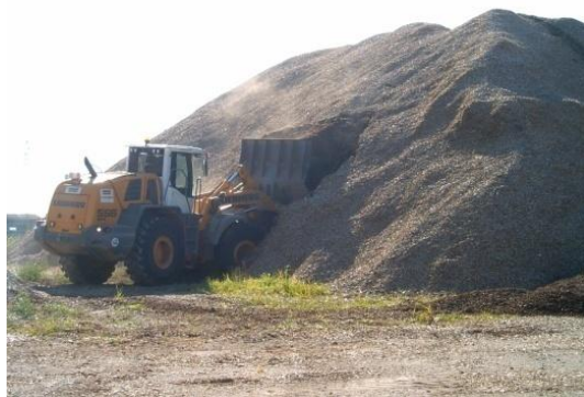
Figure 4. First section of the small-sizes pile
